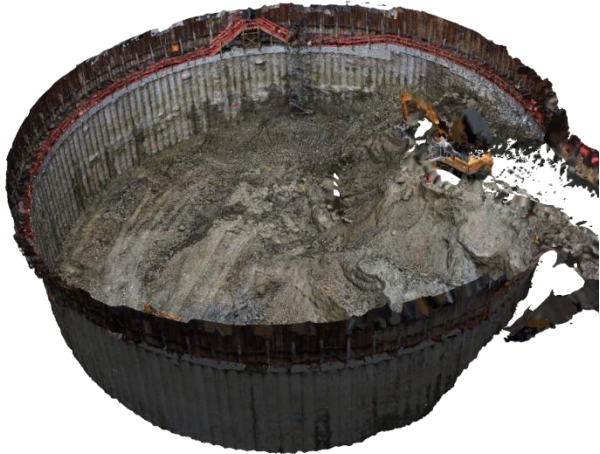
Figure 3: Point cloud of the excavation site
