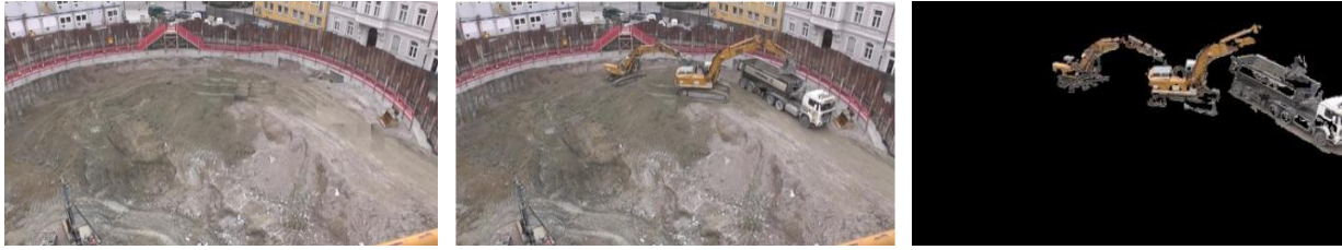
Figure 6: From left to right: sample estimated background, sample image, and foreground detection
